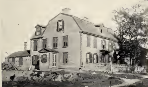
HOWE HOUSE, Willow Court.
